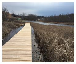
The decking is almost finished as of March 16th, and the curbing has begun from the Prescott end of the boardwalk. Railings will come next, along with other finish work.
